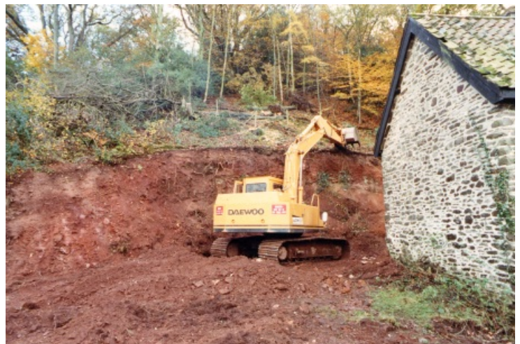
Excavating the drive area
