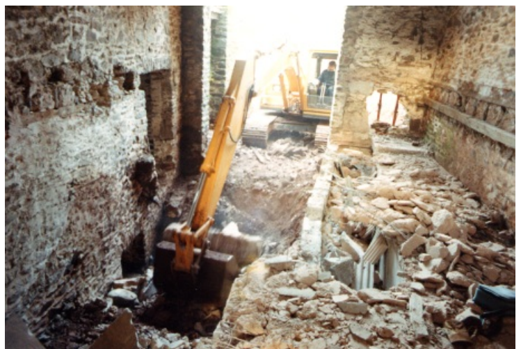
Removing the corn silo base and the rubble infill
