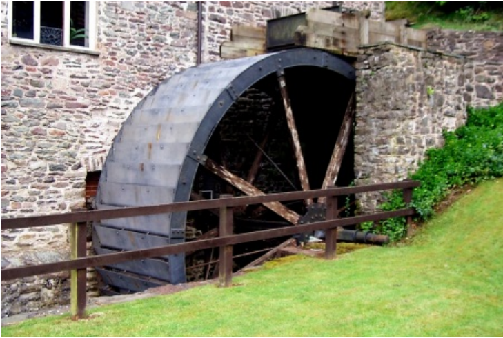
The 18 ft (5.49 m) diam. x 6 ft (1.83 m) wide overshot Water Wheel, which has 8 oak spokes each side and 56 buckets. Power was taken from the wheel by rim drive, 8 sections of gear teeth being bolted to the inside frame and driving a small pinion.
