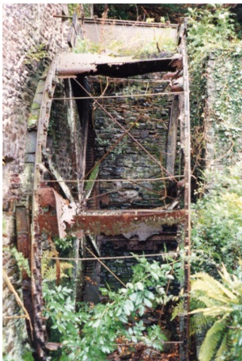
The water wheel before restoration
