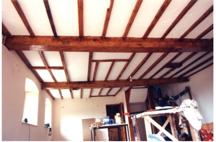
The finished ceiling retaining the old beam positions
